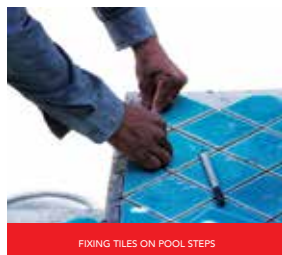
FIXING TILES ON POOL STEPS
