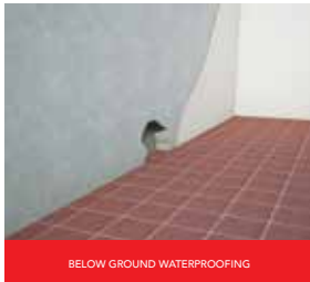
BELOW GROUND WATERPROOFING
