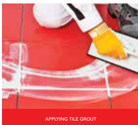
APPLYING TILE GROUT
