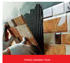
FIXING CERAMIC TILES
